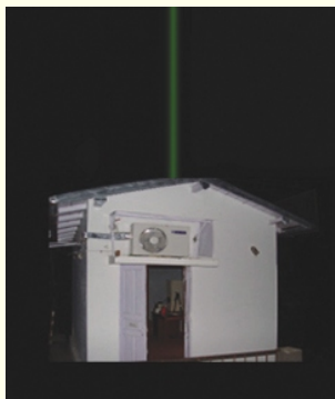
Housing where LIDAR is placed.
