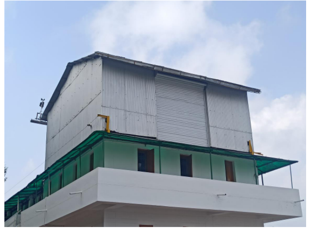
Fig. 2. (Color online) Roll-off roof structure of 130-cm DFOT.
